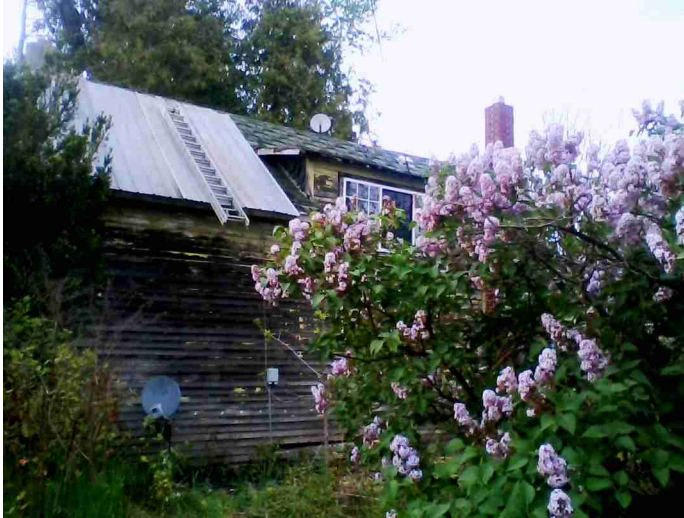
South side of the North Street Station during roof repair in the spring of 2017. The large window was installed and other modifications were made in the mid 1940's to upgrade the structure as a residence.
