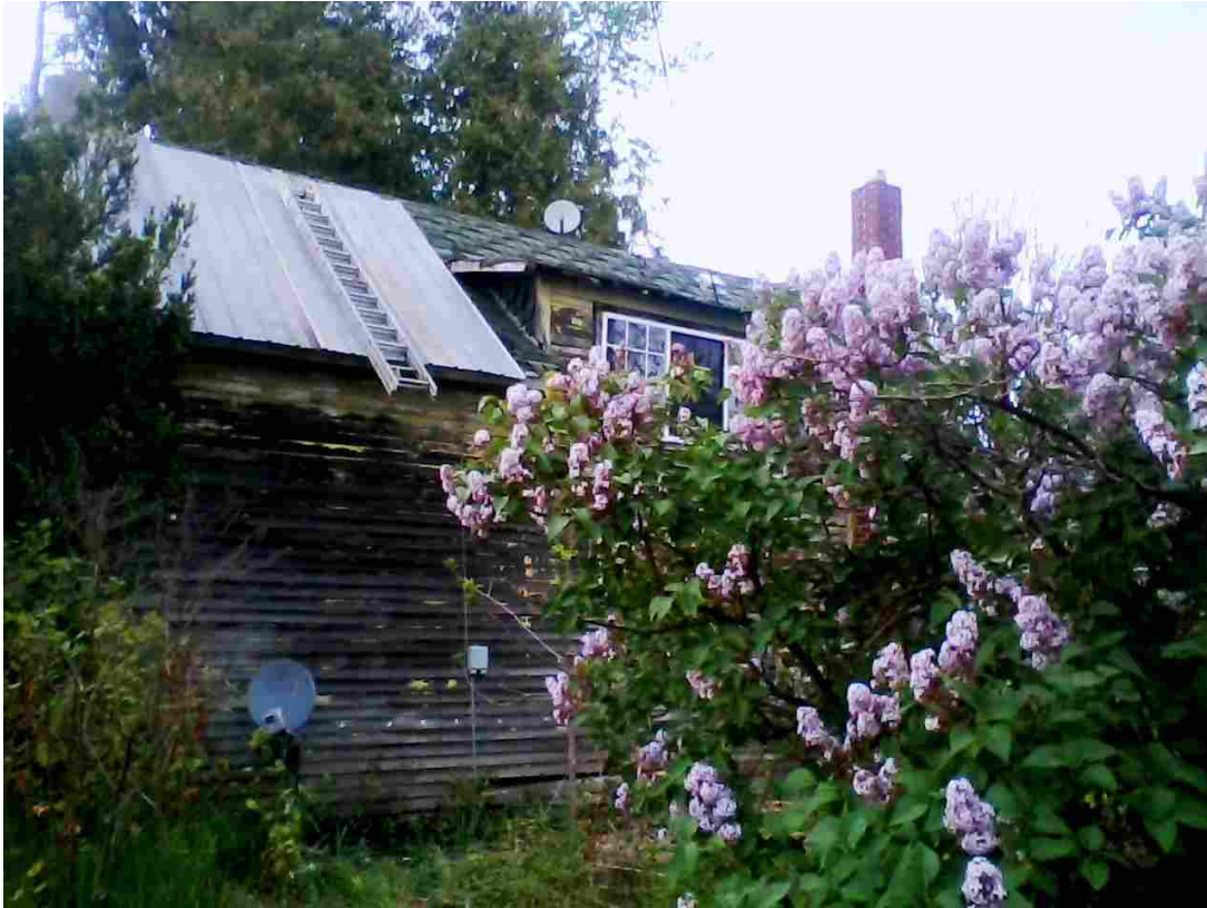
Start of metal roofing installed by TLC member Carl Hallead on 2017 May 20.
